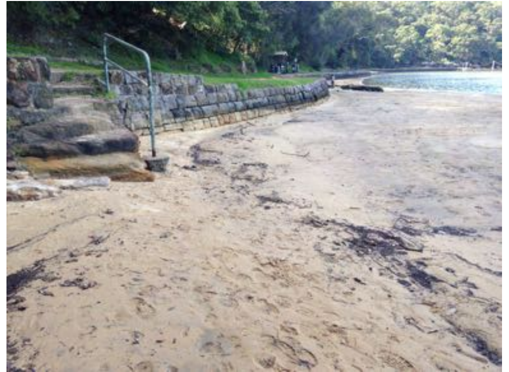
Seawalls around baths
